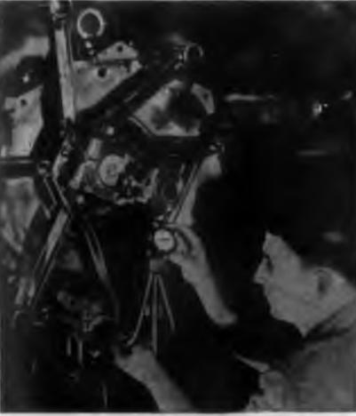
Master rod, with articulated rods, assembled to crankshaft. Silver Bearings made by Conn take the brunt of the entire power output . . . help increase speed.
