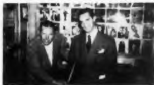
Chuck being measured for new uniform
