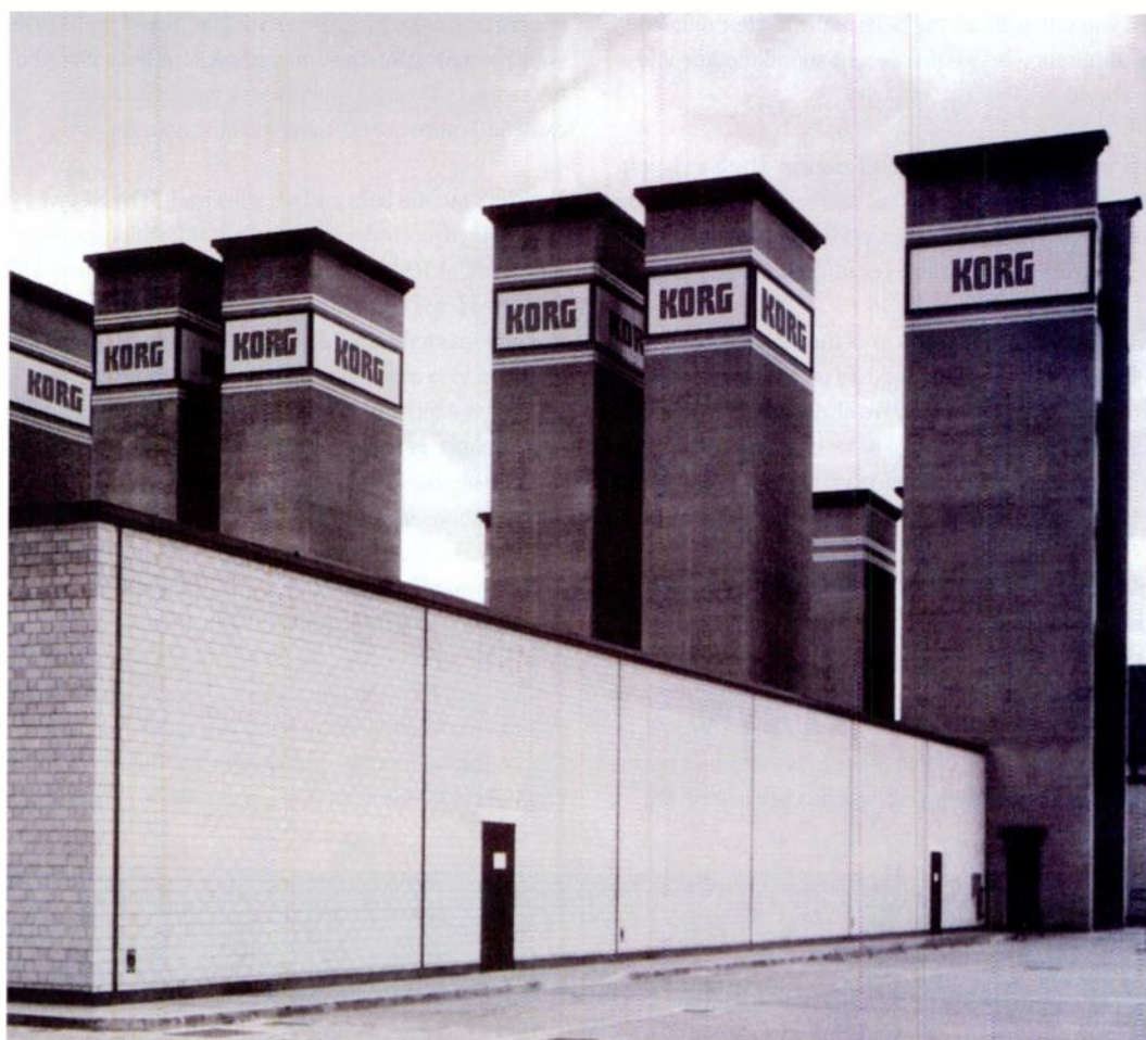
The Korg Power Plant, Long Island, NY.
