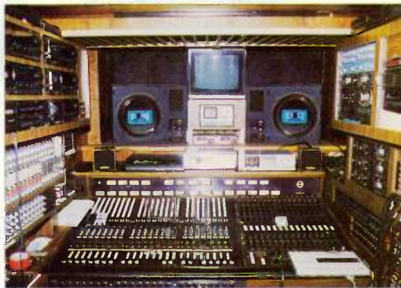
Here's a view of the monitoring area in PER's Mobile II truck.
