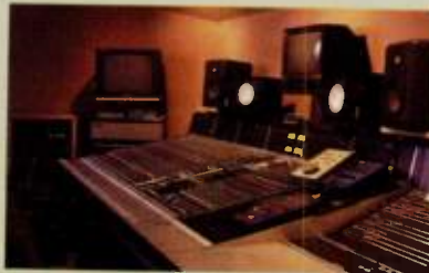
S.S.L. 4040 E/G with Total Re-call Control Room 3
