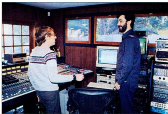
A bank of Hoffer and Petralia's outboard gear lines the wall to the right of Petralia. The rack-mount equipment includes a pair of Brent Averill—modified Neve 1073 preamps and the engineers' beloved Empirical Labs Distressors.
