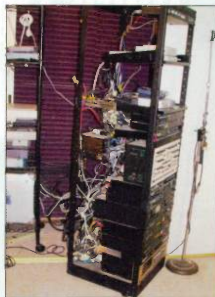
FIG. 4: You can maximize floor space by using an equipment rack on casters and leaving enough extra cable to roll it out when you need to access its connections.
