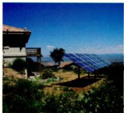
➤➤ FIG. 3: If you have the property, you can employ a ground-mount system for your solar panels.
