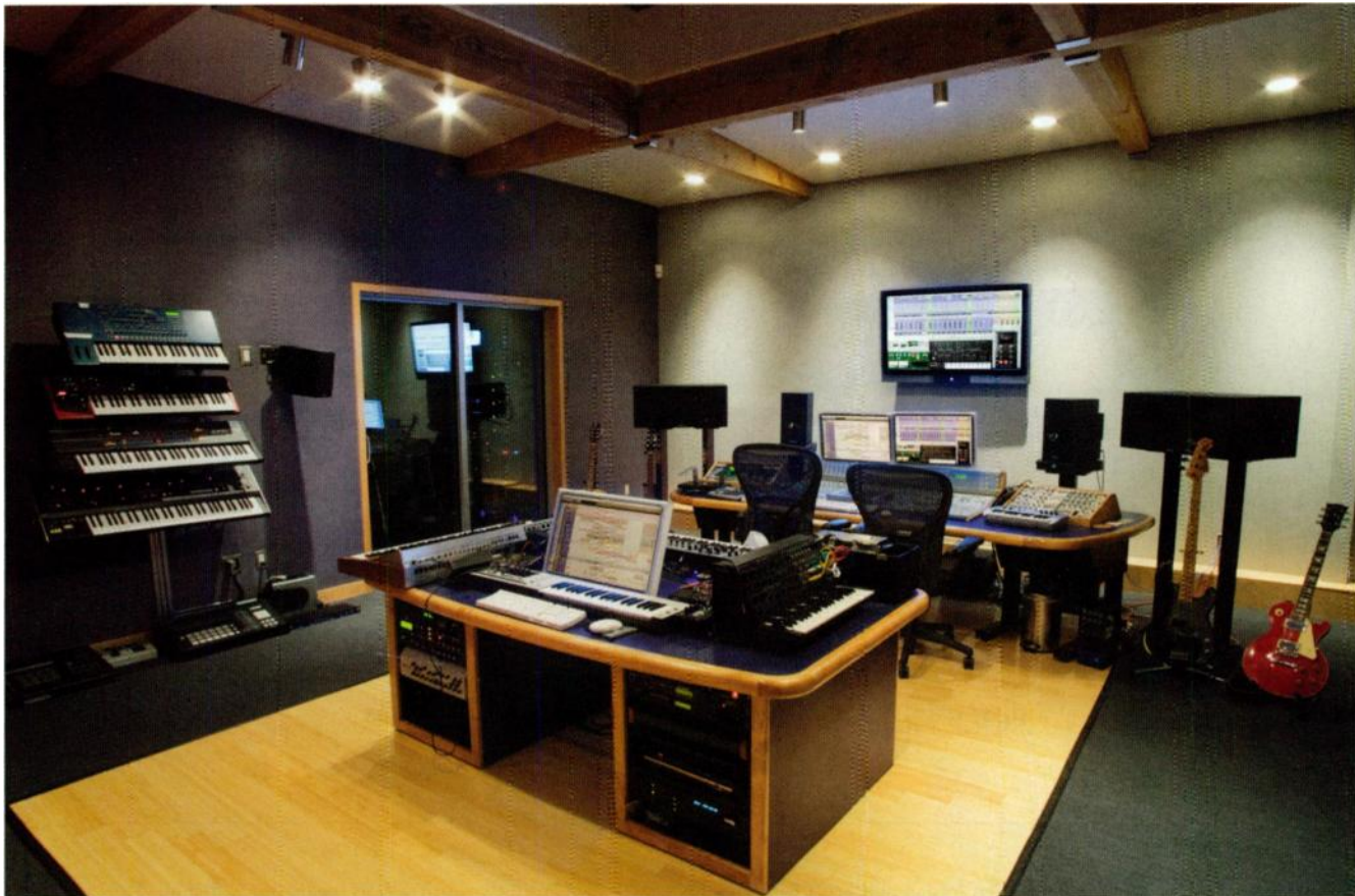
FIG. 1: A view of the Crystalwerks control room. The glass doors on the left open to the machine room.
