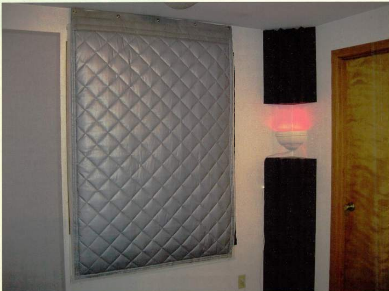
Fig. 1. Acoustics First StratiQuilt (diamond-pattern quilt) seals off a window. It's mated to the jamb with industrial velcro.
