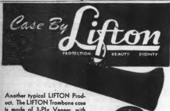
Another typical LIFTON Product. The LIFTON Trombone case is made of 3-Ply Veneer, with the unusual feature of both top and bottom (including the graceful bell shape) each constructed of one continuous piece.
