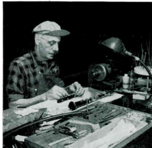
It takes seven 8-hour days to make and mount a set of oboe keys, starting with 355 tiny parts.
