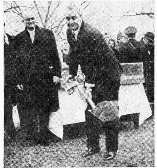
President Johnson breaks ground for the John F. Kennedy Center for the Performing Arts, with Roger L. Stevens, chairman of the Center's board of trustees, looking on.
