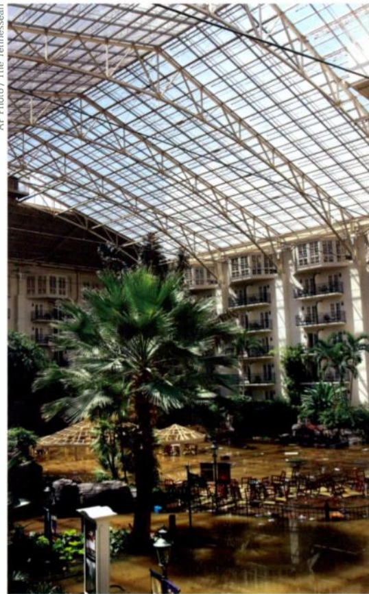
WATER FLOODS the Cascades portico of the Opryland Hotel in Nashville May 3.
