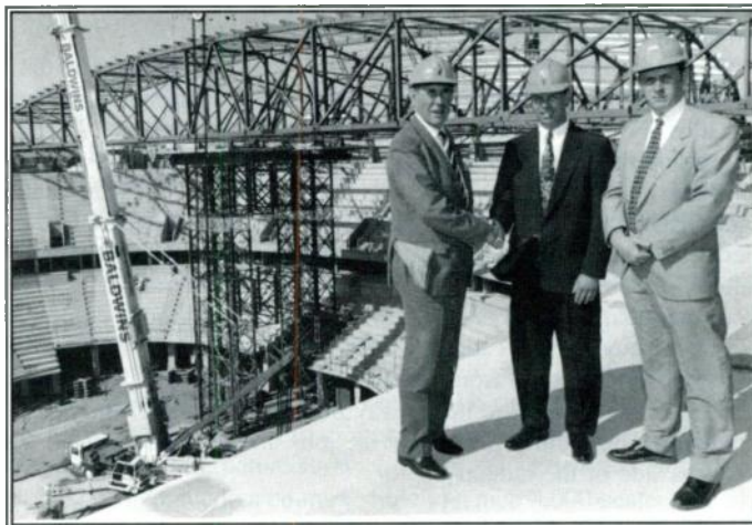
In his visit to Manchester, England July 15th, the Secretary of State for National Heritage, the Rt. Hon. Peter Brooke MP, tours the Manchester Arena construction site. When it's finished, it will be the largest multi-purpose indoor venue in Europe. (L-R) Brooke is escorted by Lee Eskilsen of Ogden Entertainment and Simon Parker of U.K. developer Vector Investments Ltd.
