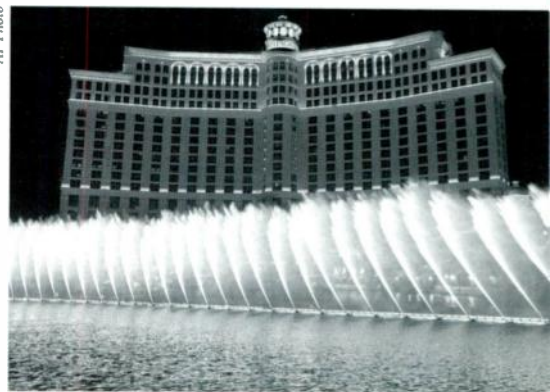
IN PREPARATION for its October 15th opening, the Bellagio Hotel tests its amazing water show in the 11 acre lake in front of the $1.6 billion Las Vegas property. The free nightly shows feature more than 1,000 moving water jets which create displays 240 feet high set to music. Said to be the most expensive hotel ever built, the Bellagio will house $300 million in art masterpieces by Monet, Renoir, Picasso, van Gogh and Matisse.
