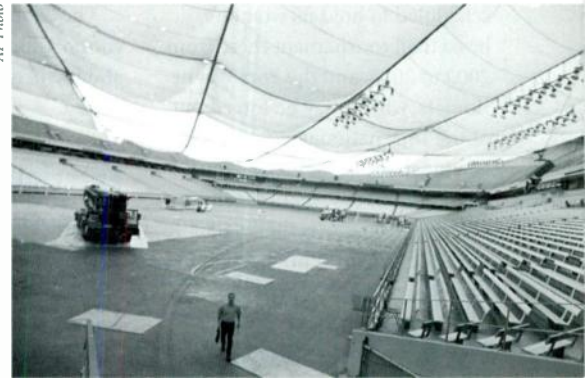
THE SKYLINE OF SYRACUSE, N.Y., looks a bit different since the 6.5-acre roof of the Syracuse University Carrier Dome was deflated. The stadium is replacing the original 64 Teflon-coated fiberglass panels installed in 1980. The $14 million project is expected to be completed in two months. Pictured leaving the facility is director Pat Campbell.
