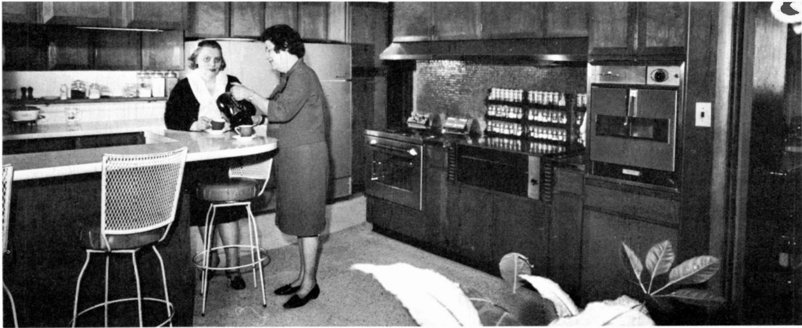
THE BACK ROOM at R. Poust & Son is this big, open kitchen that is actually the Poust family's working kitchen. It is also used for monthly cooking schools, such as are being discussed by Mrs. Ralph Poust (left) and Ruth Barr, New Jersey Power & Light home service representative. Schools are held in the evening, and no selling efforts are made.
