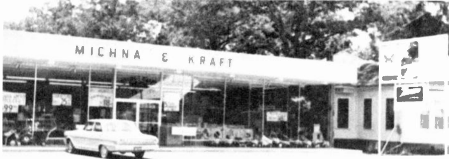
Ample parking space is provided right in front of Michna & Kraft's Firestone Store. The store has about 4,500 square feet of selling space.
