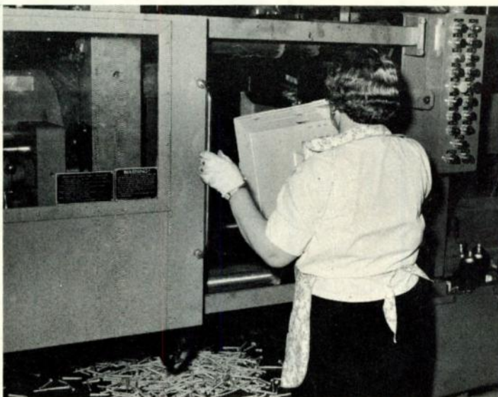
Portable tv set's plastic back is removed from machine
