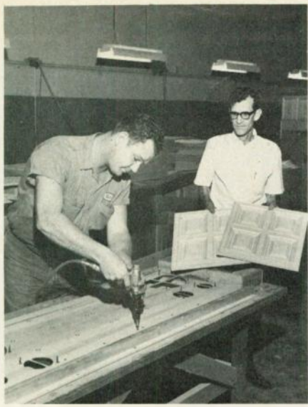
Panel is attached to plywood support
