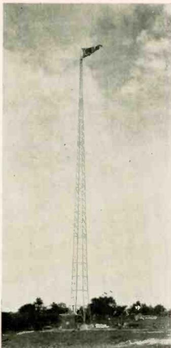
The tall lattice-work steel tower which serves as the vertical radiator for station CMQ. Photo taken during construction period.
