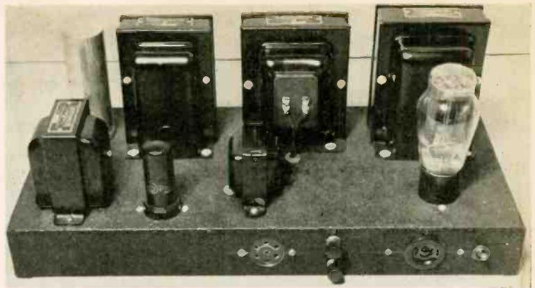
View of the combined power amplifier and power-supply chassis.
