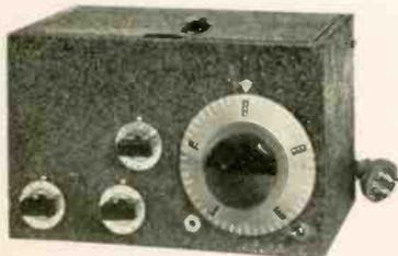
Center control is R.F. Trimmer, lower left control is Regeneration and lower right control is Audio Gain.
