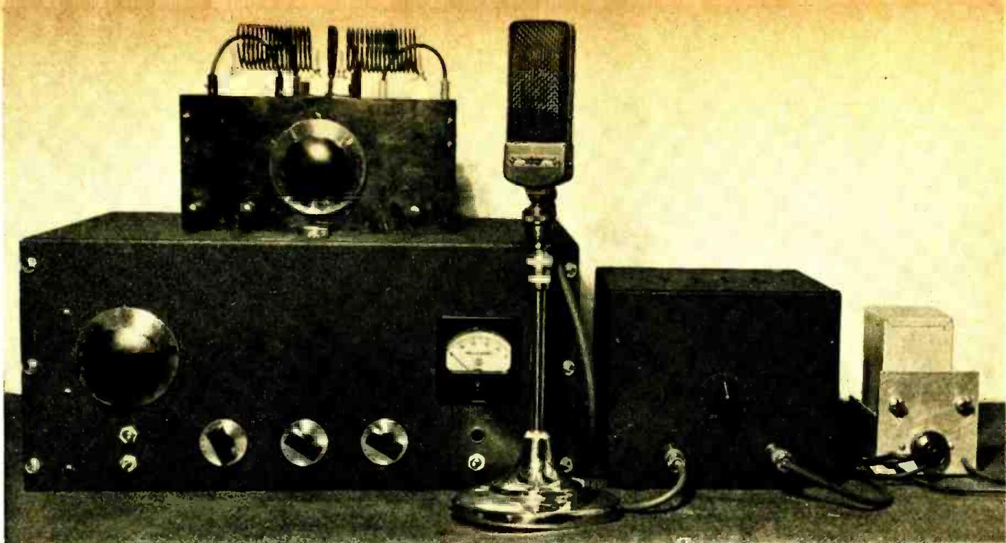
NEWCOMER'S TRANSMITTER WITH ITS PRE-AMPLIFIER AND AUXILIARY POWER UNIT, AT RIGHT, AND ANTENNA TUNING UNIT.
