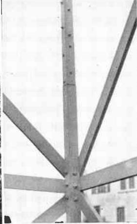
Close-up of butt-joint taken from inside of tower and showing how the 2½-in. section joins the 2-in. member.
