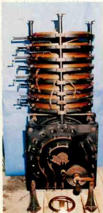
Washington Navy Yard oscillation-transformer assembly and wavechanger switch, one of the several 6' high, early spark transmitter components. (McElroy photo)
