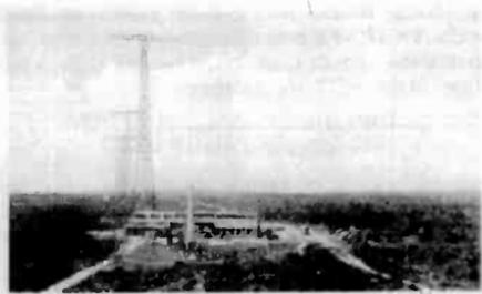
"Radio Station, Rocky Point, L.I." This is RCA's "Radio Central" which went on the air on November 5, 1921, as the Riverhead Facility. The antenna towers were 412 feet high with 150 feet cross arms. The last tower was demolished on December 13, 1977.
