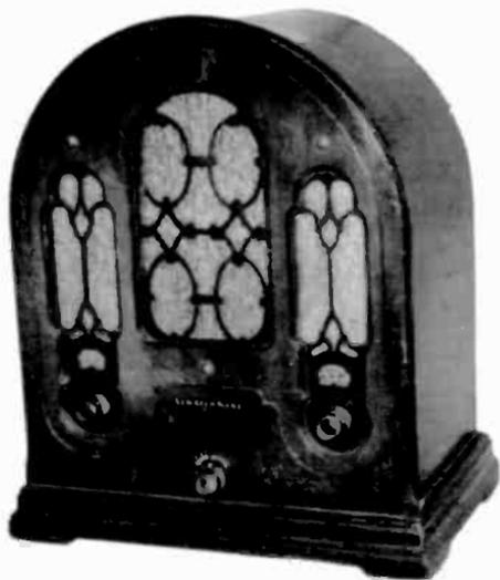
**ATWATER KENT MODEL 165** – This 5-tube superhet cathedral was produced in 1933. The thin, delicate trim around the grille cloth is very fragile and oftentimes broken. (Wally Worth – Wollaston, MA)
