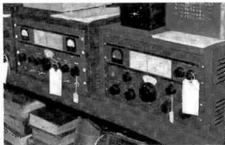
Ham gear included a Collins 32V transmitter, left, and a 75A-1 receiver, right.
