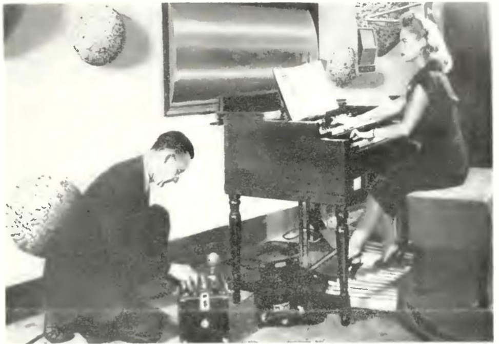
A section view of the Kasper-Gordon recording studio with acoustical-correction diffusers arranged in random pattern on one wall.
