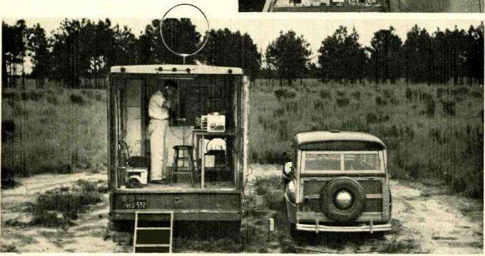
Thunder hunting equipment on location near Madison, Florida. Loop antenna on truck picks up static. The engineer in top picture is watching the indication of a directi which registers how often the static exceeds a given level.
