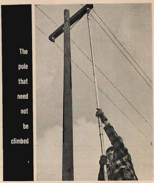
Fastening wires with new tool.
