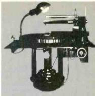
In 1939, while many turntable manufacturers were trying to make the transition from horn phonographs to electrical record players, Denon developed its first direct-drive turntable. (shown above). Denon engineers discovered that only a direct connection between motor and platter - free of the pulleys or belts found in more primitive drive mechanisms - could completely eliminate speed fluctuations that obscure musical detail.
