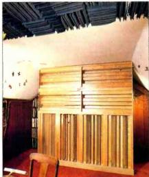
Fig. 6—The dead end of a Live End/ Dead End (LEDE) room in Pisha's home. Front speakers are B & W 801Fs and Janis W1 subwoofers.
