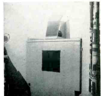
Fig. 2. Baffle installed in room corner.
