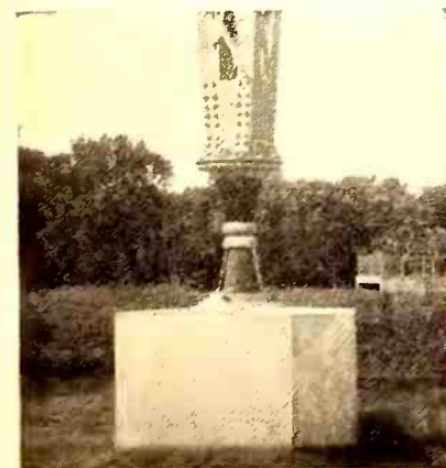
Porcelain Insulated Base with Swivel Socket
