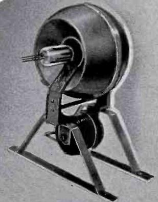
● A developmental r-f amplifier stage using the RCA-825 at 500 Mc. The photograph shows the resonator, the tube, the electromagnet and general arrangement of parts. In use at RCA Communications, Rocky Point, Long Island, N. Y.
