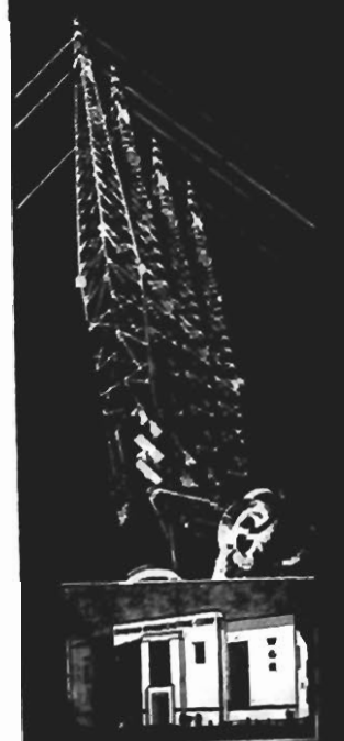
New $350,000 Transmitter Plant BUFFALO BROADCASTING CORPORATION
