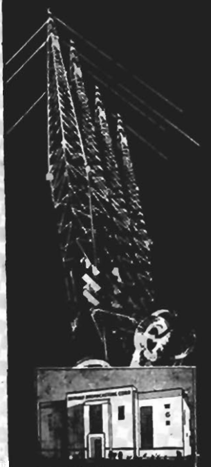
New $350,000 Transmitter Plant BUFFALO BROADCASTING CORPORATION
