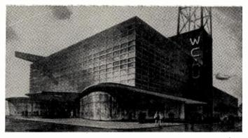
RADIO AND TELEVISION center planned by WCAU Philadelphia is pictured in architect's drawing above. To include a four-story main building of limestone and stainless steel, the \$2,000,000 structure will be headquarters for all WCAU operations upon completion.
