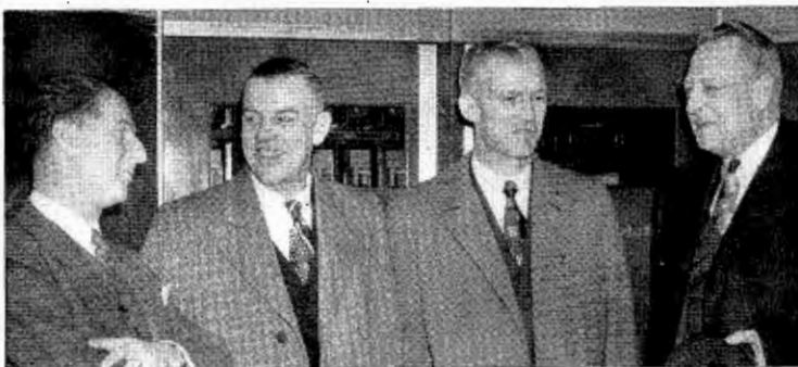
ATOP the O'Sullivan Bldg. tower, Baltimore's highest structure, members of FCC inspect transmitter of WMAR-TV, Sunpapers station. (L to r) Commissioner George E. Sterling; Sunpapers vice president and radio director, E. K. Jett, who was succeeded on FCC by Mr. Sterling; Commissioner Rosel H. Hyde; and Sunpapers vice president and executive editor, Neil H. Swanson, who has sparked newspaper's TV programming.
