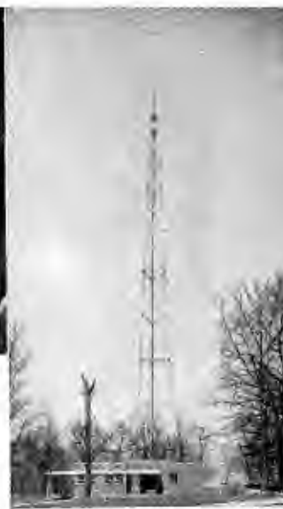
GRACEFUL tower and antenna of WSIX-FM Nashville rises to 292 feet, and is on a hill 1,110 feet above sea level. Station, owned by WSIX Broadcasting Co., increased its radiated power to 7 1/2 kw April 9.
