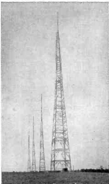
▲ Four sturdy Blaw-Knox towers support WNAO's TV, AM, and FM antennae. A 12.5 kw FTL transmitter feeds a Federal TV antenna.
