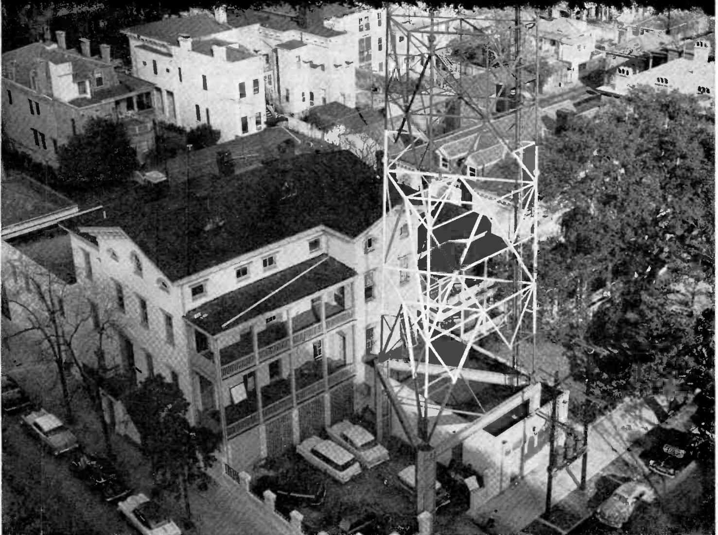
**JOB DATA:** Station WTOC-TV, Savannah, Ga. Self-supporting Ideco tower, 501 feet including 12 bay antenna, 40 lb. wind load. Transmitter building partially surrounds steel frame base for tower.
