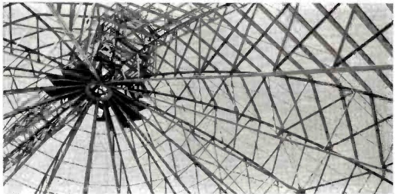
**Steel Spider Web.** If you ever needed it, here's proof that amazing things can be done with steel. This is an 83-foot-high dome for a potash storage building that will be covered with steel sheets. This complicated structure was *prefabricated* and erected by American Bridge Division of U. S. Steel.
