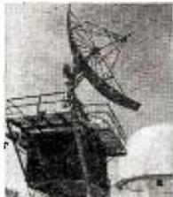
Microwave antenna tower typical of those used in systems built for the Ohio Turnpike and the Illinois Toll Road.
