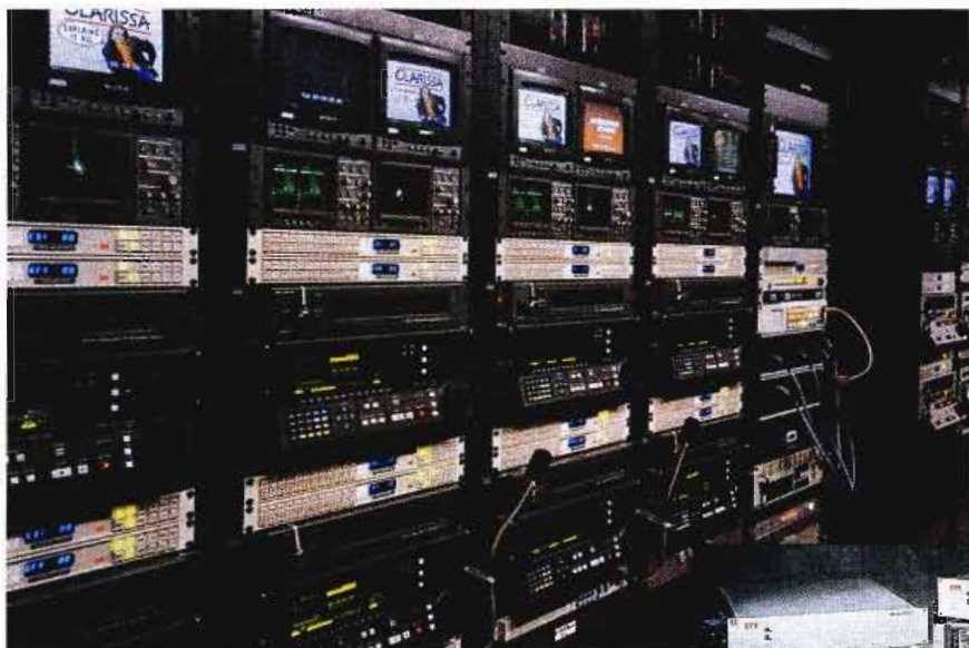
Perpetual transformation will continue to characterize the television plant beyond the "digital era." Racks of VTRs like these D-2 machines will ultimately yield to "digital video servers." The BTS Media Pool (r) provides time-scalable (10 minutes to hundreds of hours) video recording using RAID technology. In time, these systems will be low-cost enough to replace VTRs in most playback and distribution applications.
