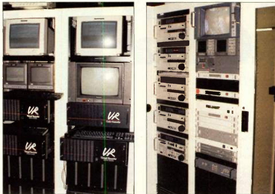
At WOFL Orlando, Odetics Spectrum multichannel automation software is managing a hybrid storage/playback network that uses both digital disk recorders (l) and conventional tape decks (r).
