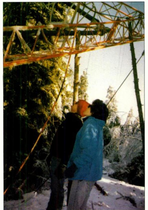
Fred Miller, vice president of programming, Dudman Communications, and Marth Dudman, president/general manager, survey the fallen tower of WEZQ(FM) Bangor, Me.
