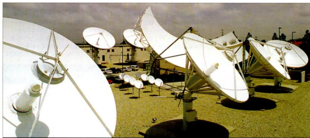
DirecTV's uplink farm in Denver transmits digitally compressed content into orbit 22,300 miles from Earth.
