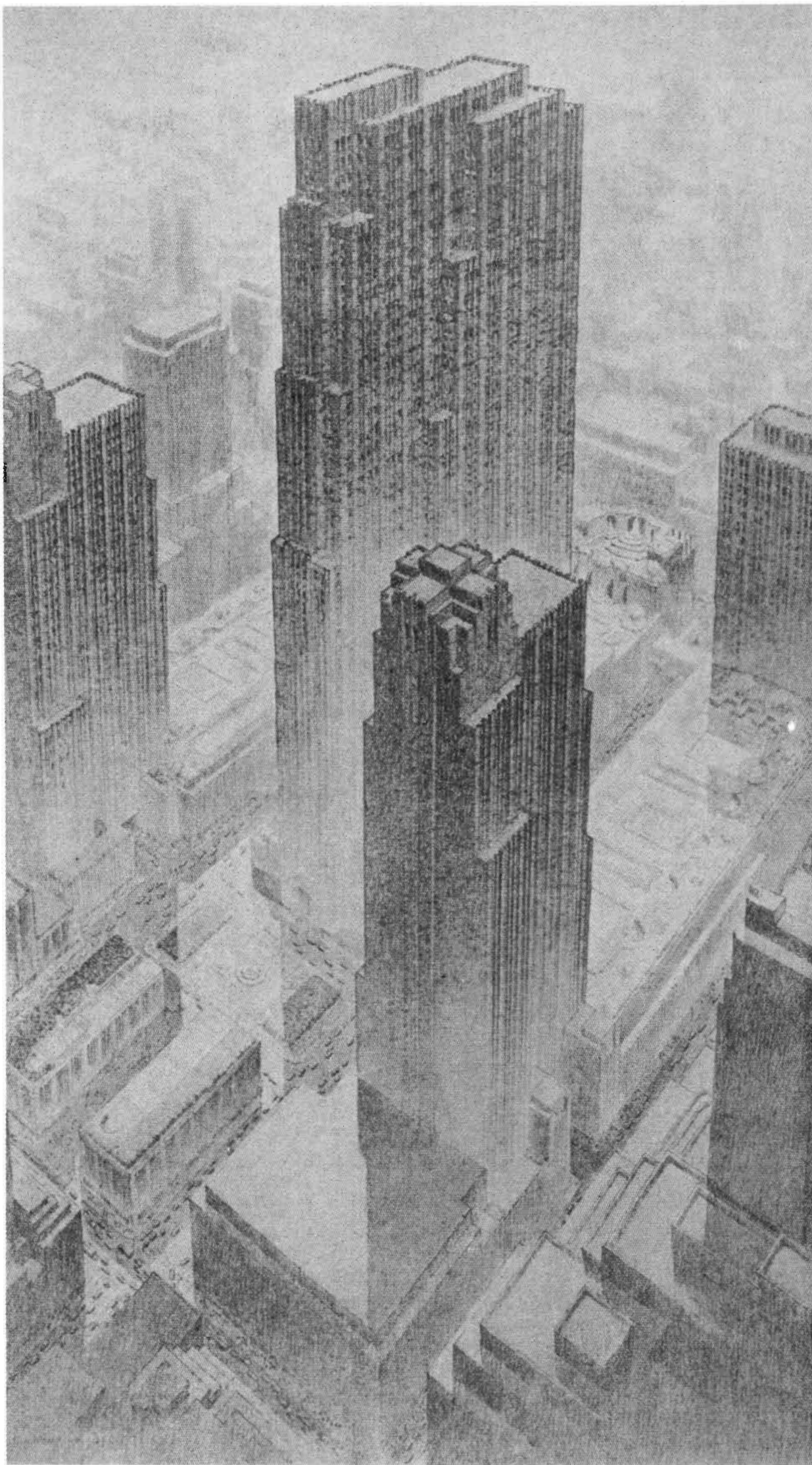
RADIO CITY—An air view of the general development that will cover three square blocks from 48th to 51st Streets, between Fifth and Sixth Avenues, New York City. The view is from the east side of Fifth Avenue. This $250,000,000 building project, the greatest in modern history, is being financed by John D. Rockefeller, Jr.
