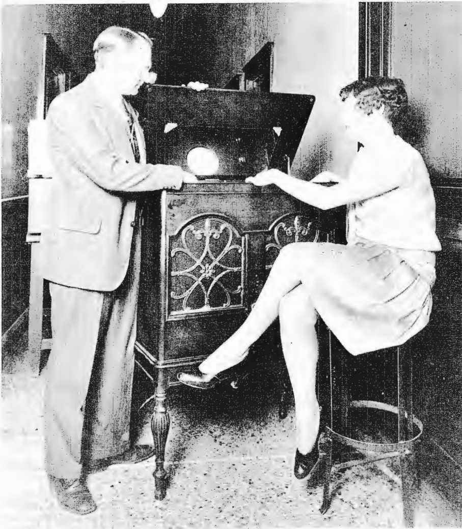
The tube cometh. Experimental television was well on the way by the time BROADCASTING began reporting the electronic media in 1931, thanks to the groundwork of such pioneers as Vladimir K. Zworykin, shown here (in 1929) demonstrating a new cathode ray TV system he developed at the Westinghouse Research Laboratories. The Russian-born scientist applied for a patent on an electronic beam television pick-up tube in 1923. Politics was first in line. These General Electric television cameras, from wgy Schenectady, were said to be involved in the first TV remote when they covered New York Governor Al Smith accepting the Democratic presidential nomination in 1928.
