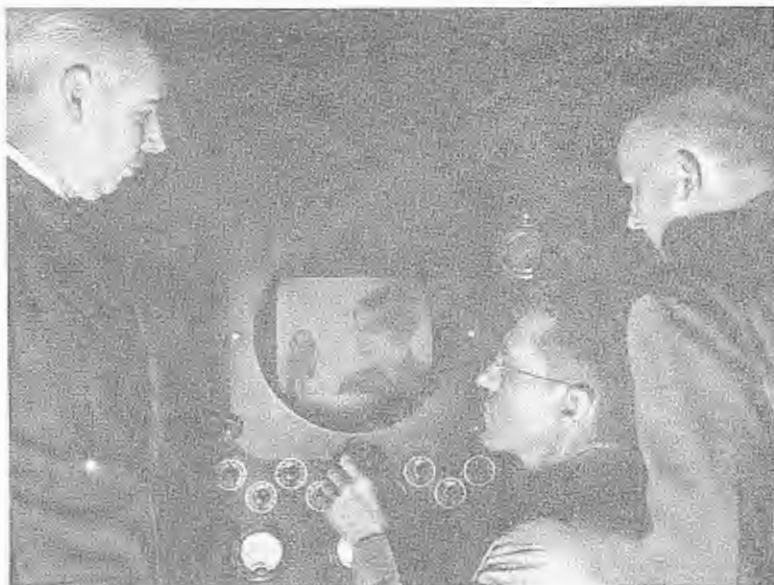
BEFORE the monitor panel at a demonstration by Midland Television Inc. at KMBC, Kansas City, Arthur B. Church (left), president of KMBC and a principal stockholder of Midland, J. R. Duncan, chief television engineer, and G. L. Taylor, president of the company, study the 441-line television image of Caroline Ellis, who begins Caroline's Golden Store for General Mills, Minneapolis, on WHO, Des Moines, Aug. 15.
