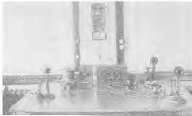
EQUIPMENT here is the proud development of General Electric Co. and actually worked, aided by collection of batteries under the table. One of the telephones apparently was used as a microphone. Old timers on engineering staffs will recognize some of the paraphernalia.
