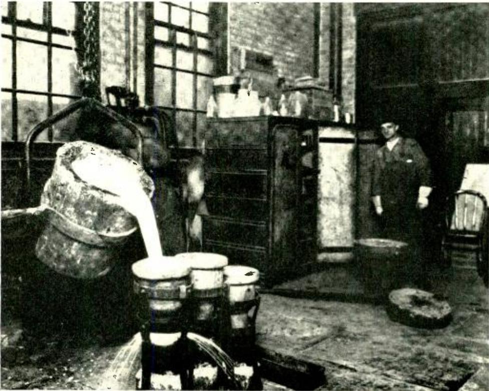
*Fig. 3—Casting permalloy into ingots suitable for later crushing and grinding*
