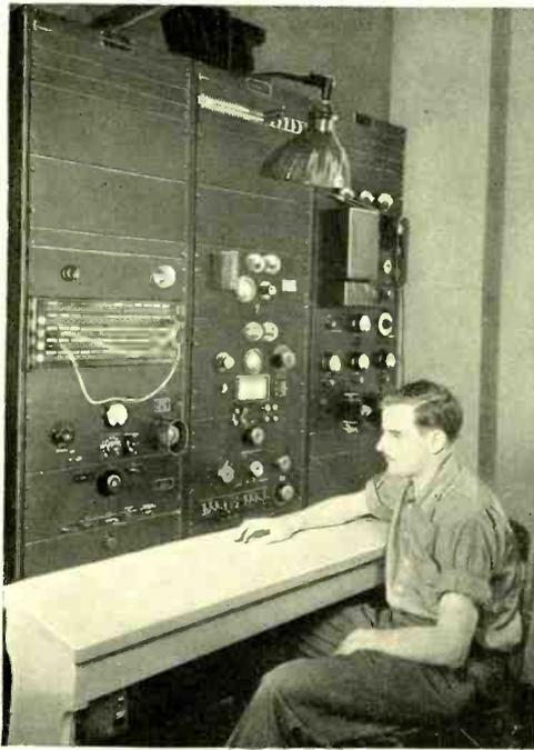
*Fig. 5—Testing equipment is used each morning for transmission measurements on each channel*
