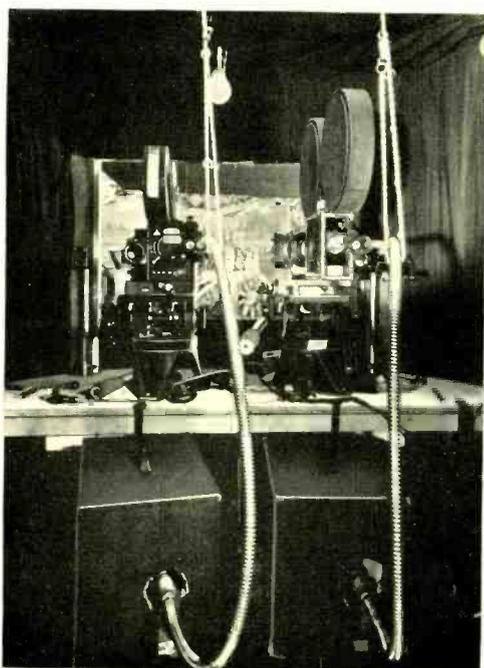
*Fig. 3—Development of silent cameras is in progress to remove the necessity of placing the cameras in these sound-proof booths, and thus to regain the camera freedom of the silent pictures*
