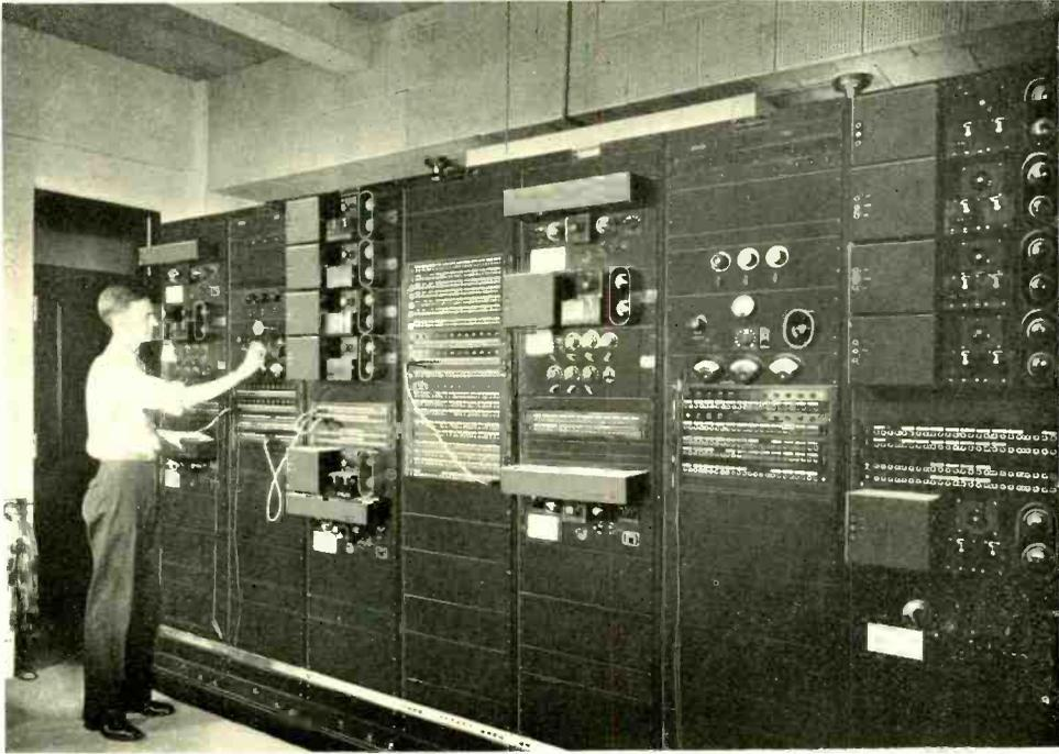
*Fig. 4—In the United Artists' installation, amplifiers (of three bays for each channel) are mounted in pairs, with the members of each pair separated by a patching bay*
