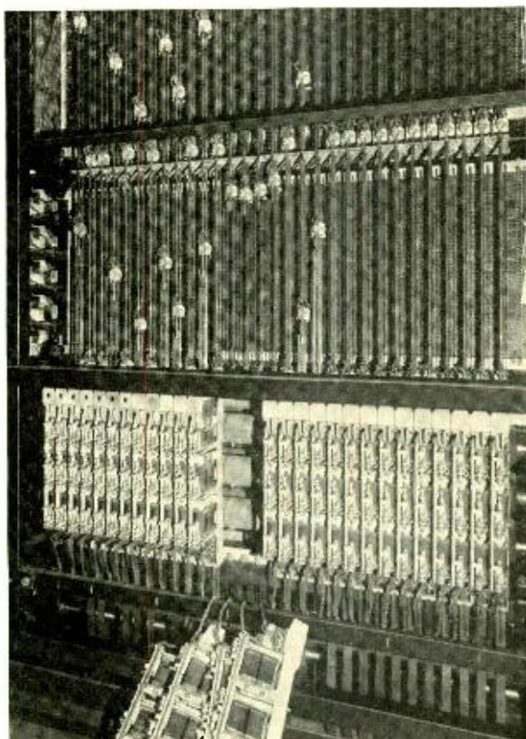
*Fig. 1—A selector frame has space for thirty elevator rods on one side. Three of the clutches have been laid back to show the cork rolls*
