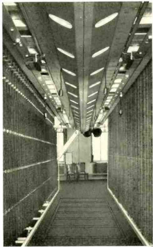
Fig. 3—Lighting for main frames combining in a very satisfactory manner high intensity with freedom from glare
