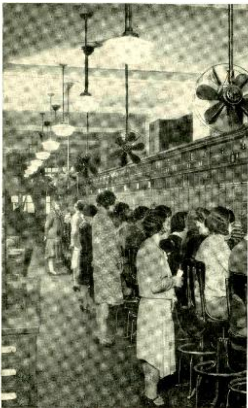
Fig. 1—An operating room in the Walker-Lispénard Building showing the new semi-indirect lighting units
